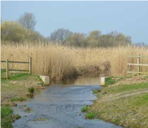
Marton Mere Overflow Channel
